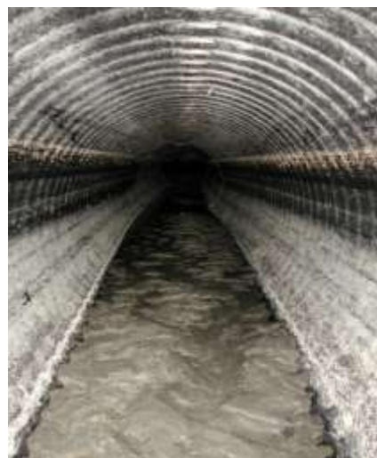
Fig. 1. Inside of a five-foot diameter drainage pipe. Sediment has accumulated on the bottom of this drain as a result of erosion from ditches leading to it. Photo by Donald Merhaut.
